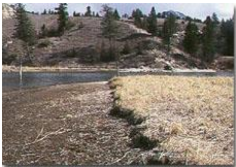
Figure 3: View east of the erosion along the bank of the Columbia River.
