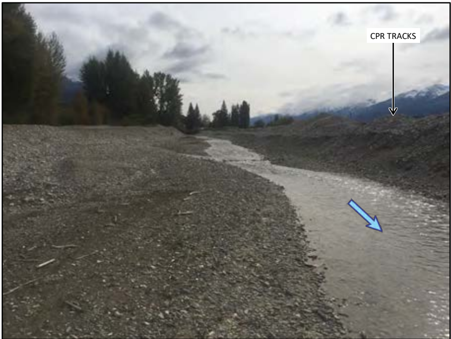
Photo 38 - September 28, 2019: Channel 300 m downstream of 14 Street culvert. In this area, Canadian Pacific Railway has dredged the channel and used the dredged material to construct training berms on both sides of the creek.
