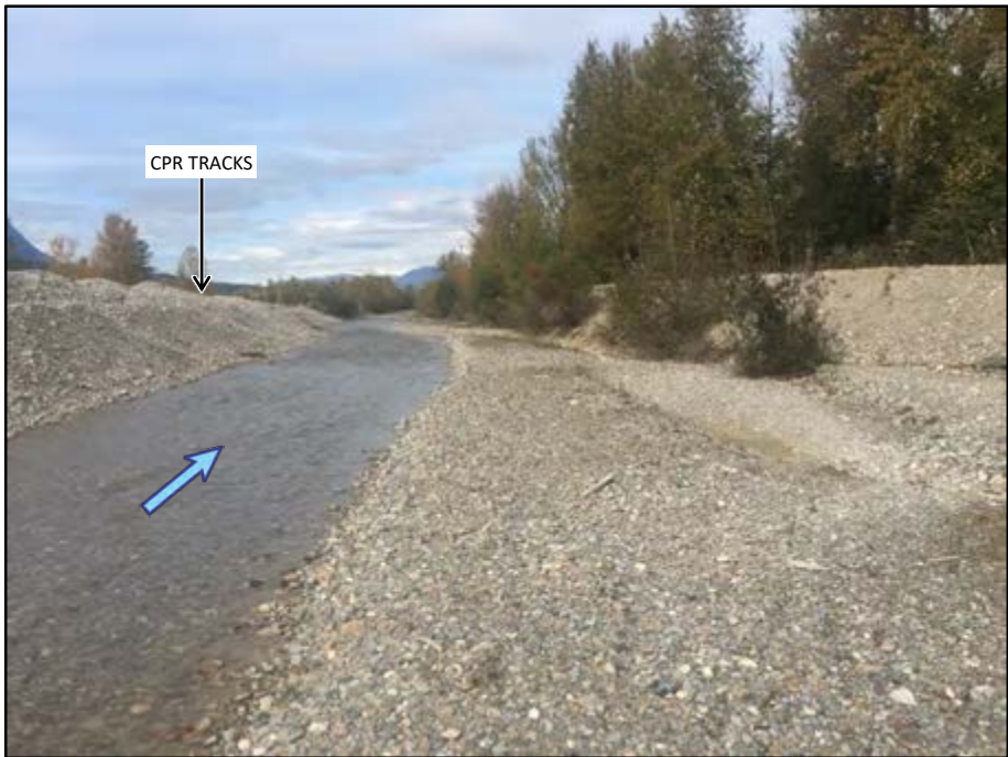
Photo 39 - September 28, 2019: Channel 300 m downstream of 14 Street culvert. In this area, Canadian Pacific Railway has dredged the channel and used to construct training berms on both sides of the creek.
