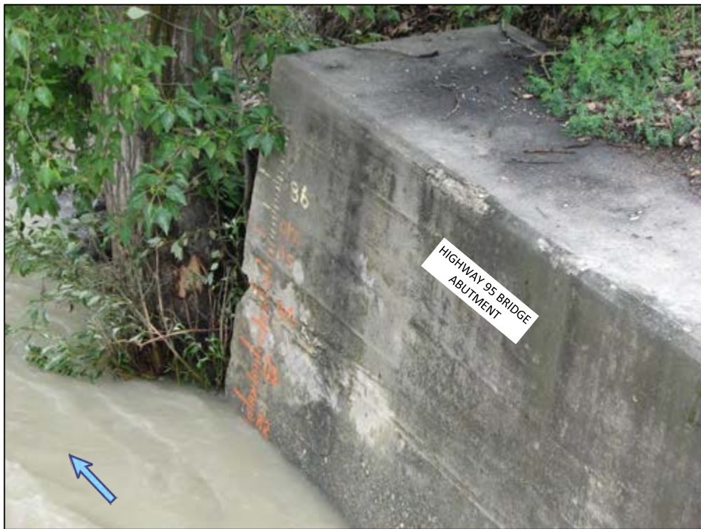
Photo 29 - June 9, 2012 (2+192): Water level at Highway 95 bridge abutment during the flood of 2012 (highest since 2007). Peak water level occurred about 3 days before photo was taken.
