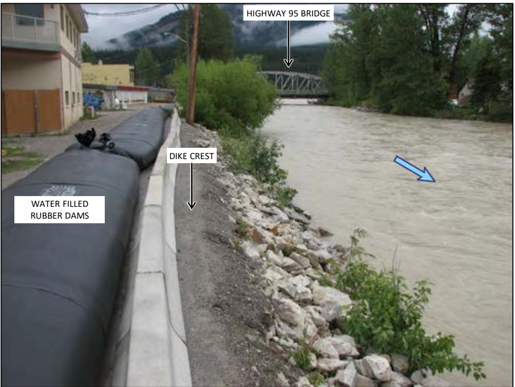
Photo 28 - June 9, 2012 (2+100): Flood of 2012 (highest since 2007). Peak flow of 352 m 3 /s was reported by the Water Survey of Canada, which occurred about 3 days before photo was taken (June 6). The Town installed barriers and water filled rubber dams to mitigate potential flooding of the historical downtown. Peak water level compared to the dike crest was observed by Town staff on June 6 and used to validate the hydraulic model.
