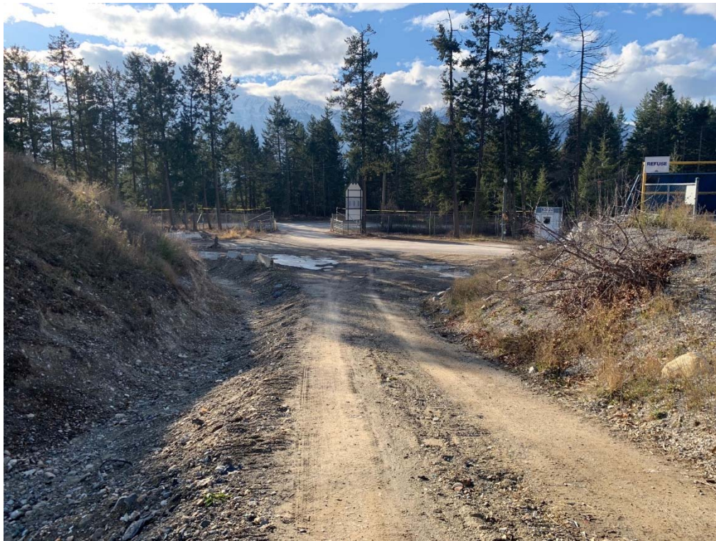
Photo-10: Internal ditches near z-wall and inlet to Western Infiltration Gallery, cleaned up and re-shaped.
