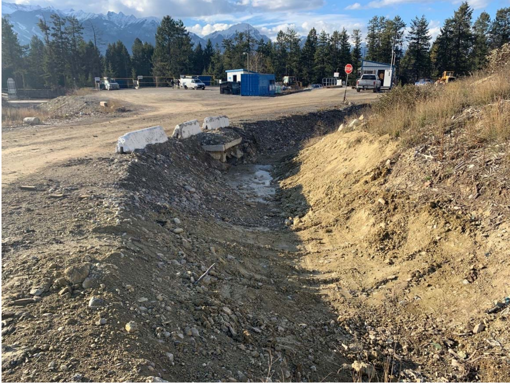
Photo-9: Internal ditches near scale shack, cleaned up and re-shaped.
