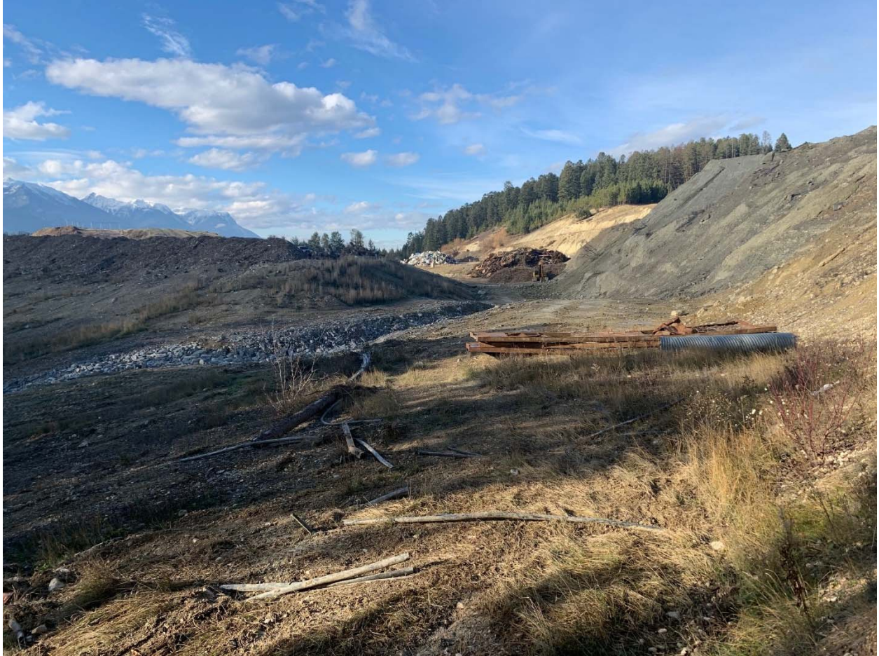
Photo-11: Photo taken from SE corner of site looking north with active borrow area on the left and Phase 1 to the right. With ever changing geometry and drainage paths in the borrow area, as cover and intermediate soils are extracted, onsite contractor is to maintain positive drainage along toe of borrow area directing run-on to the Southern Infiltration Gallery.
