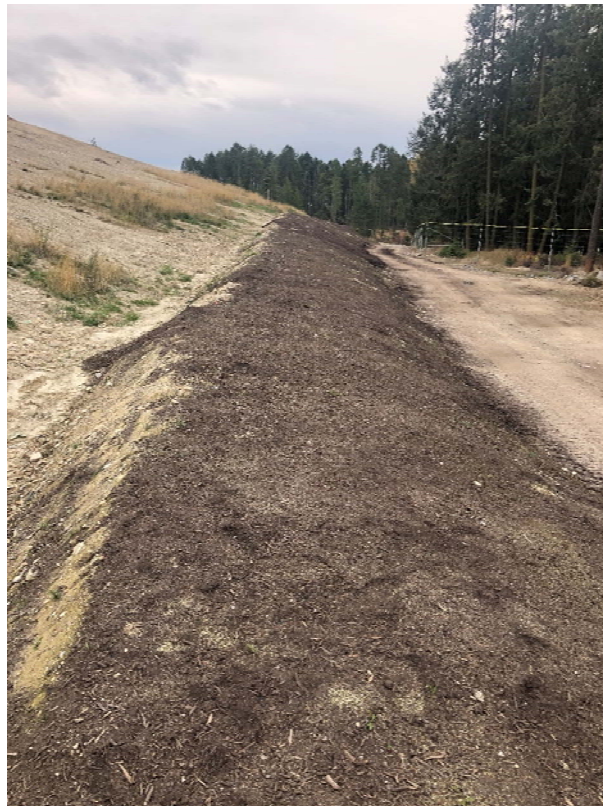
Photo-8: Western run-off control ditch directing stormwater to both the Western and Southern Infiltration Galleries. Outer side slopes of ditch received an application of topsoil and seed.
