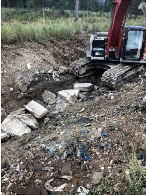
Photo-3: Infiltration key-trench being backfilled with owner supplied recycled crushed concrete in Southern Infiltration Gallery
