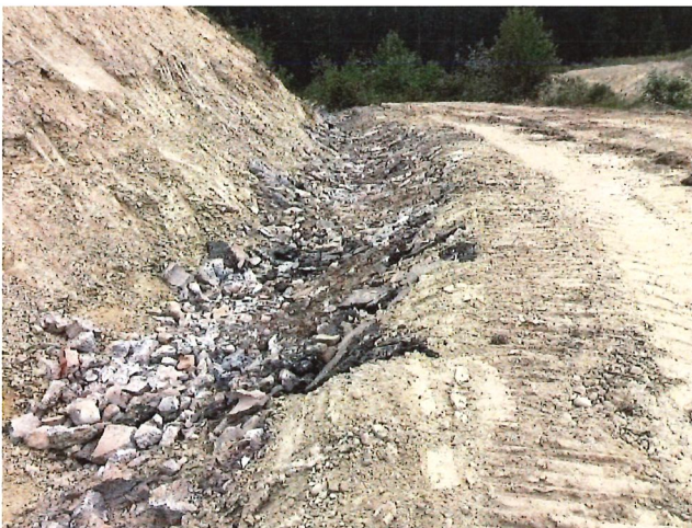
Photo 2 – Armoring of North Access Road Ditch utilizing onsite recycled products.
