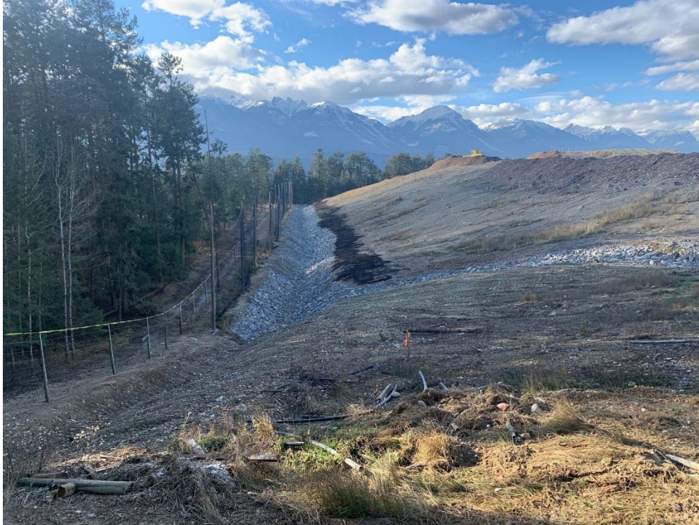
Photo-5: Completed Southern Infiltration Gallery with armored run-on and inflow ditching. Photo taken from SE corner of site, looking west.
