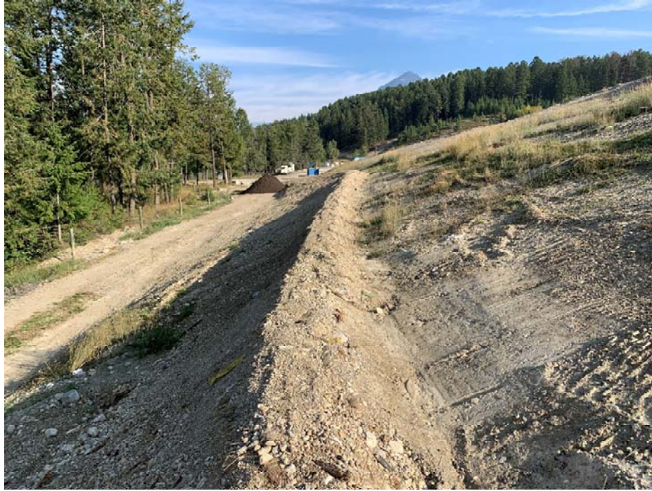
Photo-7: Western run-off control ditch directing stormwater to both Western and Southern Infiltration Galleries, pre topsoil and seeding.
