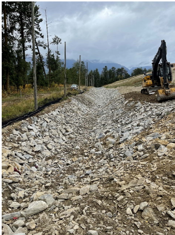
Photo-4: Southern Infiltration Gallery completed with 150-300mm rip rap and topsoil being applied to south toe of Phase 1. Photo taken from east, looking west.
