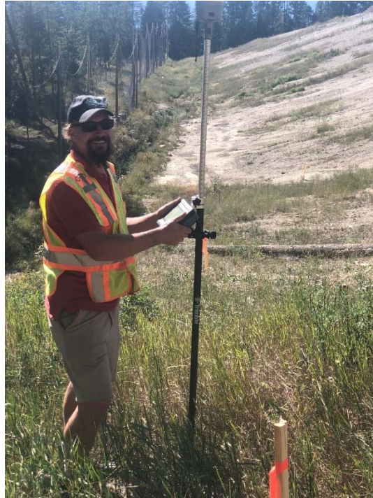
Photo-1: CSRD staff completing design layout of infiltration galleries and ditches
