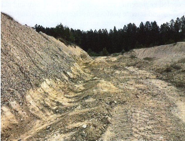
Photo 1 – North Access Road – Ditch geometry re-establishment to design specifications – this work was completed in 2022.
