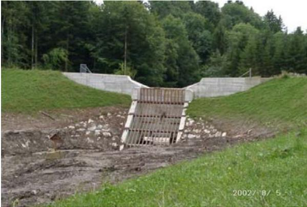
A) Looking downstream at concrete slot barrier with inclined steel rack embedded within earth fill berm (Fischbach, Thalgau, Salzburg, Austria; photo from Hübl et al., 2005).
