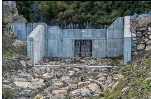
B) Looking obliquely downstream at stilling basin with concrete wing walls, concrete counter-sill and armoured bottom covered by sediment (Kleine Melchaa, Giswil, Switzerland; photo Sept. 2015 by Christian Imfeld, giswil.ch).
