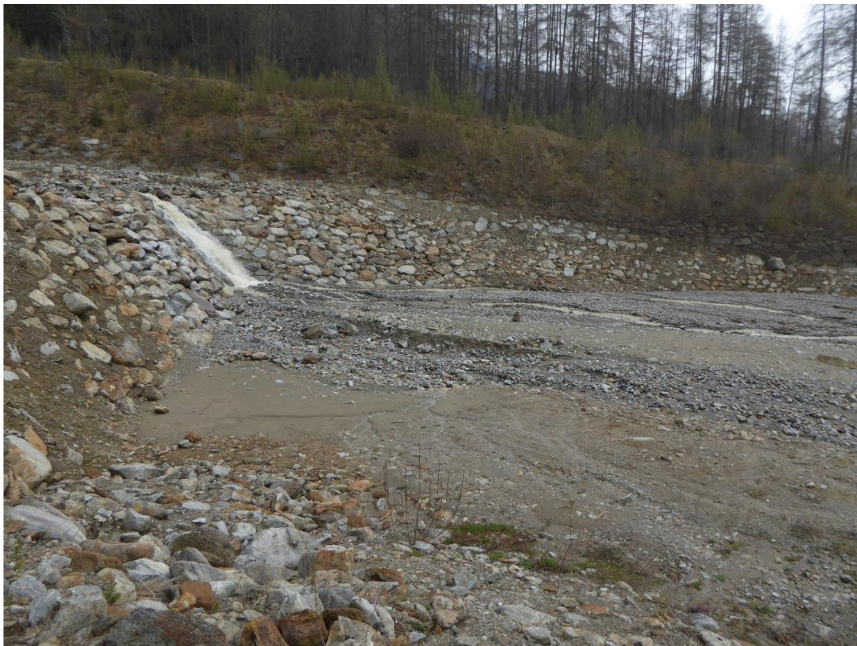
**Figure 6-1 Example of basin inlet ramp lined with grouted stone pitching (Photo courtesy of J. Hübl BOKU).**
