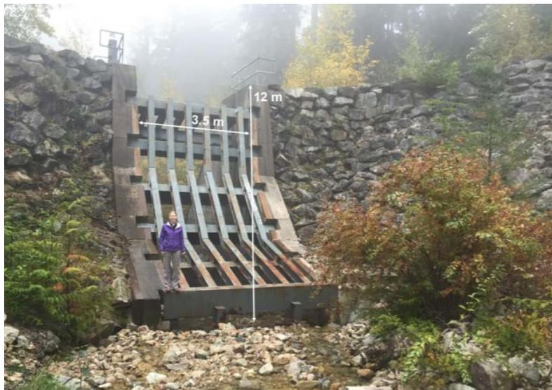
C) Looking downstream at concrete slot barrier with inclined steel rack embedded within earth fill berm at McKay Creek in North Vancouver, BC (photo from Moase, 2017).
