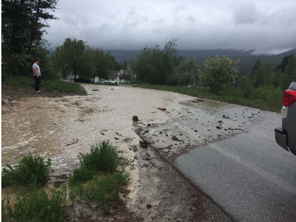
**Figure 3-9. RDEK image of Cold Spring Creek at Fairview Drive downstream of Highway 95. The culvert is not visible to the left of the road and water is flowing down Fairview Drive. May 31, 2020, 3:45 PM.**
