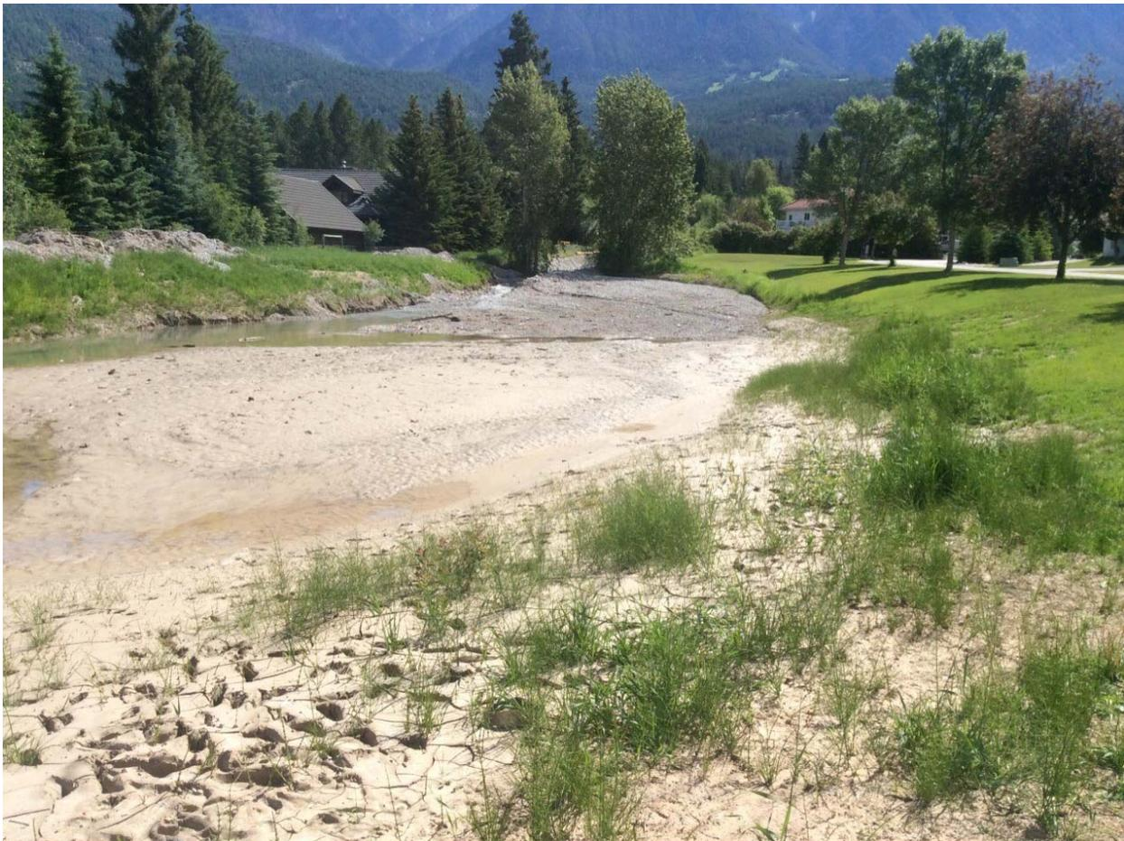
**Figure 3-16. Sedimentation pond upstream of golf course culvert on Cold Spring Creek, looking upstream. BGC photo taken June 2020.**
