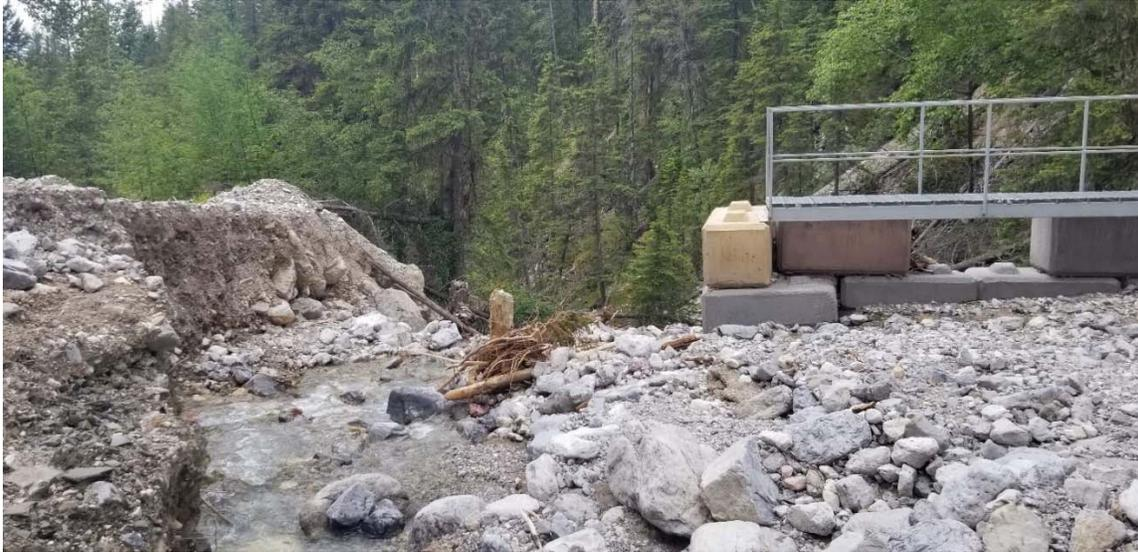
**Figure 3-5. Destroyed path across Cold Spring Creek at an elevation of approximately 1285 m, looking downstream (west). The structure likely failed through outflanking on the left (south) which subsequently eroded the foundation of the lock blocks and leading to their toppling downstream. Photo: BGC July 14, 2020.**
