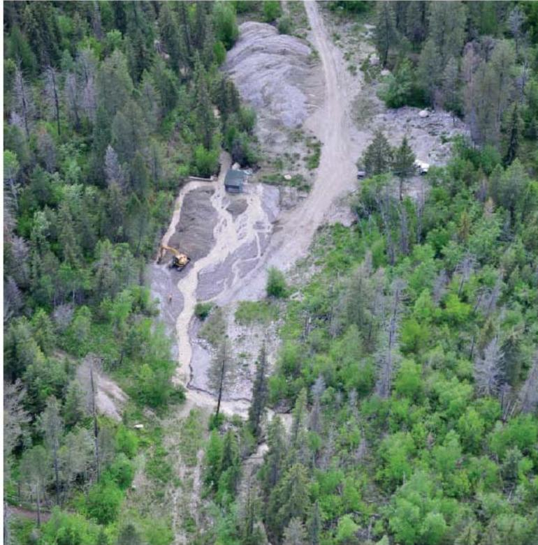
**Figure 3-7. Sediment removal after the May 31, 2020 debris flood on Cold Spring Creek. Photo: NHC, June 1 or 2, 2020.**
