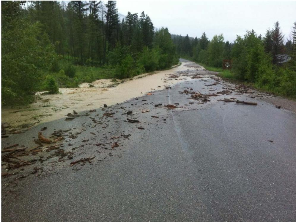
**Figure 3-1.** View upstream (east) on Fairmont Resort Road at approximately the crossing with Hot Springs Road showing muddy water and debris from an avulsion at the uppermost culvert beneath Fairmont Resort Road. RDEK photograph of June 20, 2013 7:00 AM.
