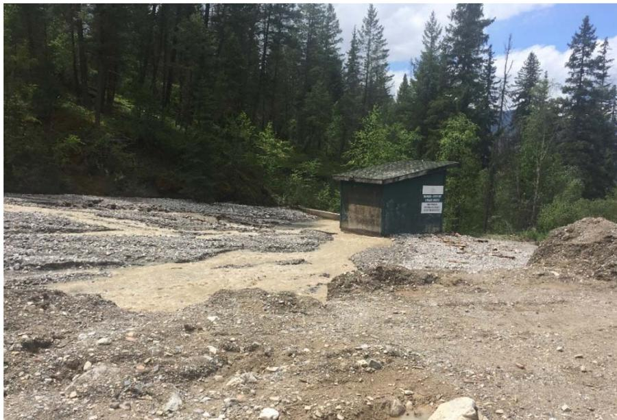
**Figure 3-8. RDEK image of the Cold Spring Creek reservoir dam entirely filled with sediment. Note that debris also overtopped to the right of the structure which is shielding the spillway from view. June 1, 2020.**
