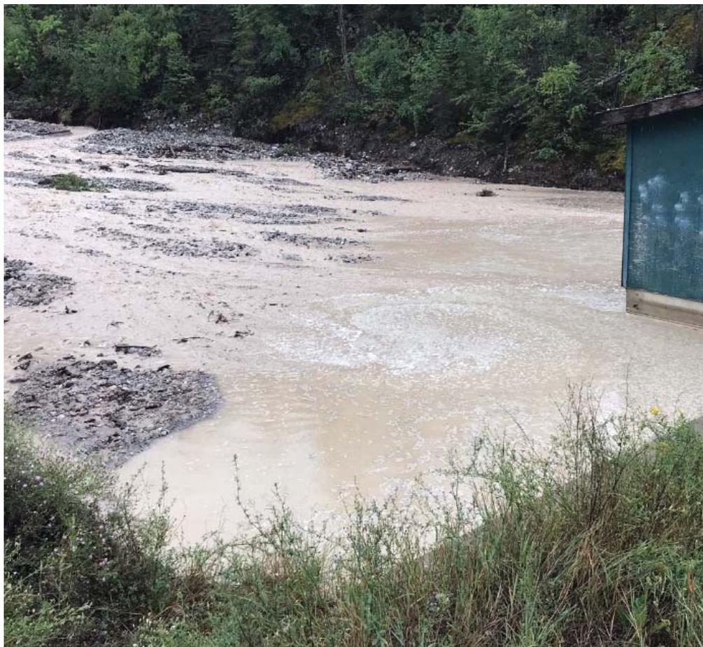
**Figure 3-4. Cold Spring Reservoir shortly after the August 12, 2020 debris flood showing the reservoir full of sediment. Photo: RDEK.**
