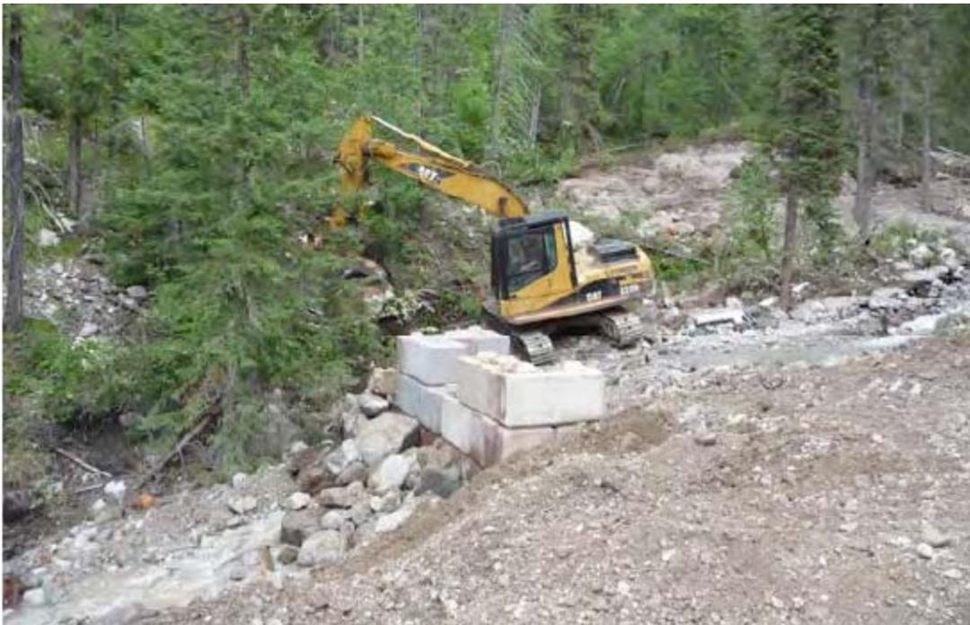
**Figure 3-6. RDEK photograph of the reconstruction of the FHSR after the 2012 debris flood (photo date unknown). This is the same location as in the previous photograph.**
