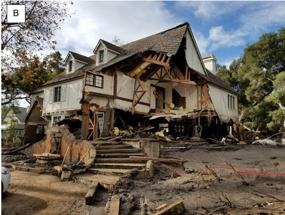
**Figure 5-1. Damage by the January 9, 2018 debris flow at Montecito, California of homes impacted with an approximate impact index of  $> 10 \text{ m}^3/\text{s}^2$ . Flow depth appears to have been approximately 2 to 3 m. Photo: Courtesy Jason Kean, United States Geological Survey.**
