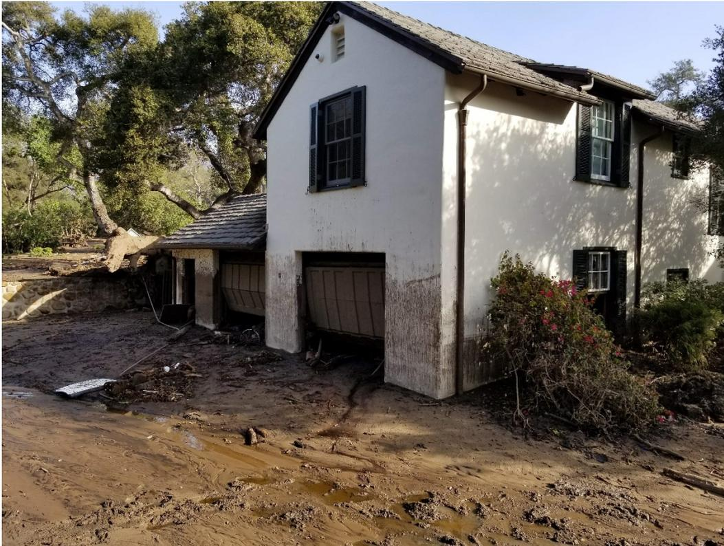
**Figure 5-3. Damage by the January 9 Montecito debris flow, California at a home impacted with an approximate impact index of < 3  $\text{m}^3/\text{s}^2$  and a flow depth of approximately 1.2 to 1.5 m. Image: Courtesy Jason Kean, United States Geological Survey.**
