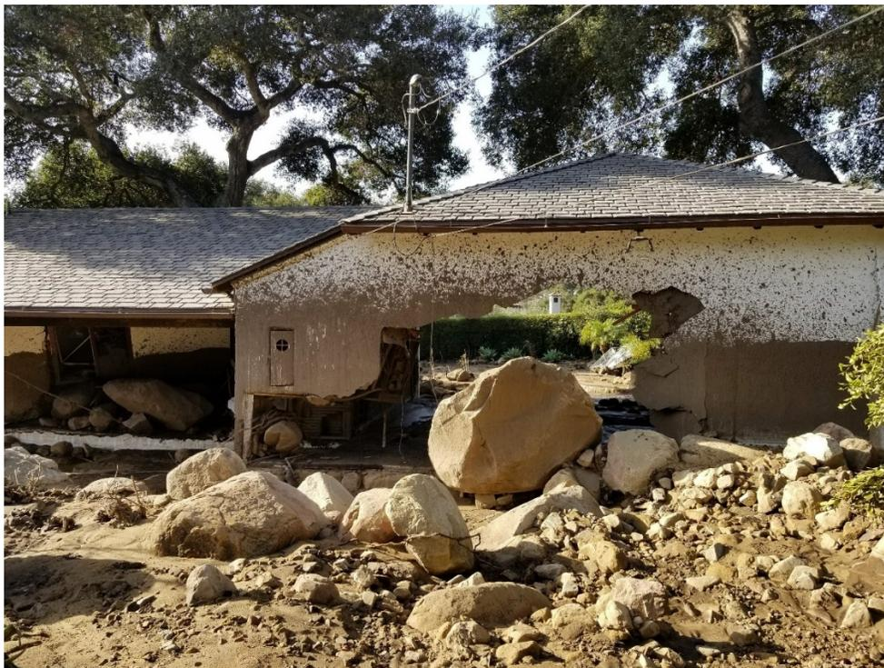
**Figure 5-2. Damage by the January 9, 2018 debris flow at Montecito, California at a home impacted with an approximate impact index of 3 to  $10 \text{ m}^3/\text{s}^2$ . Flow depth appears to have been approximately 1.5 m. Photo: Courtesy Jason Kean, United States Geological Survey**
