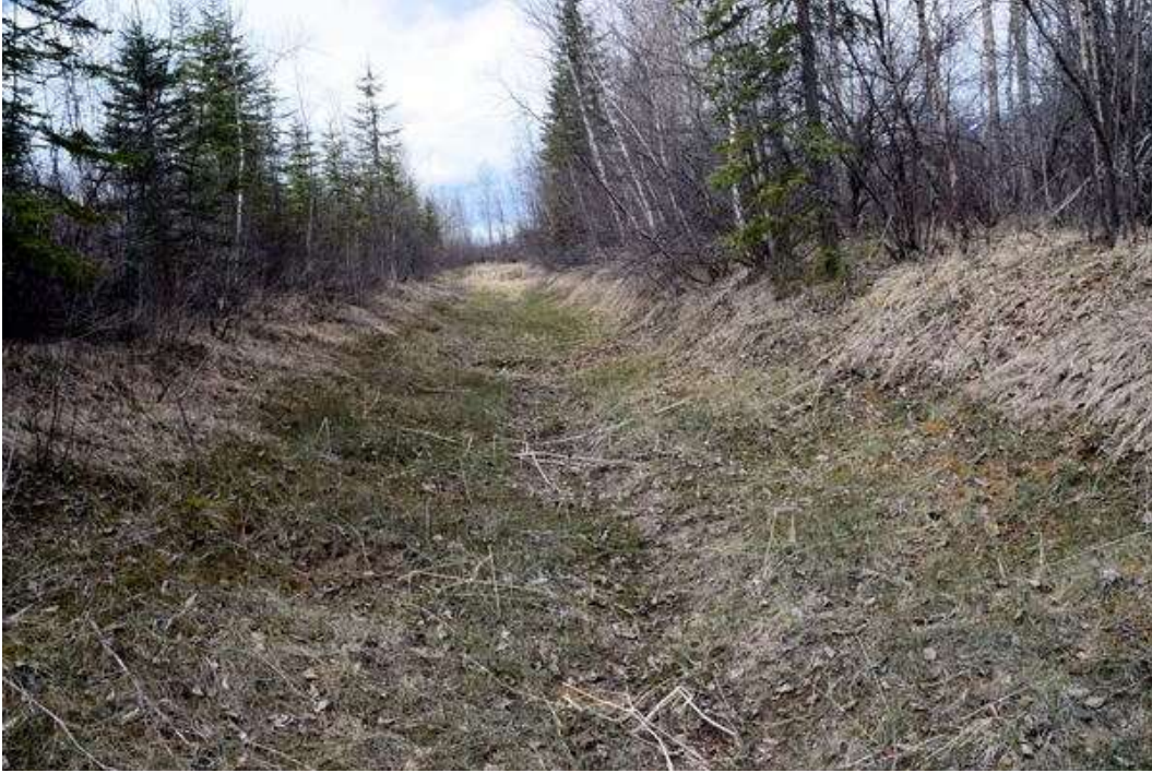
Figure 53. Here is another borrow pit ditch located along a constructed dike. The majority of the borrow pit ditches are dry because water is soaking into the ground and flowing under the dike towards the Columbia River in organic, sand, and gravel layers. The borrow pit ditches remove standing water and lower the elevation of groundwater over the entire Burges James Gadsden Provincial Park.
