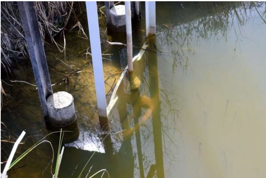
Figure 121. Leaking valves on water control structures are draining Moberly Marsh.
