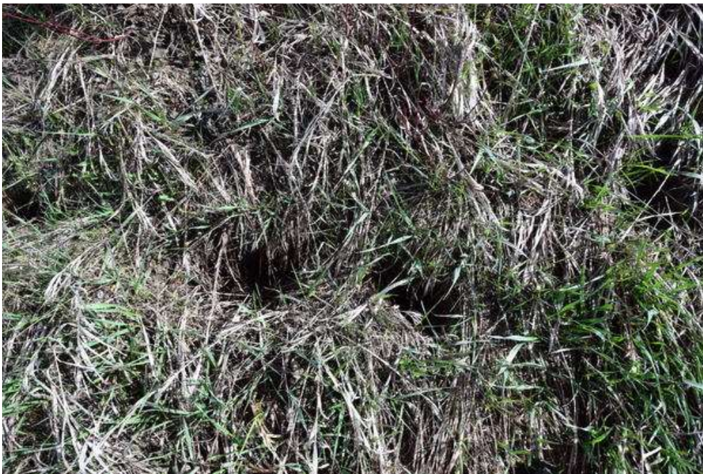
Figure 45. The holes are collapsed muskrat burrows in an interior dike on the Sime Compartment. Muskrat and beaver burrowing activity have caused breaching and failure of interior dikes.
