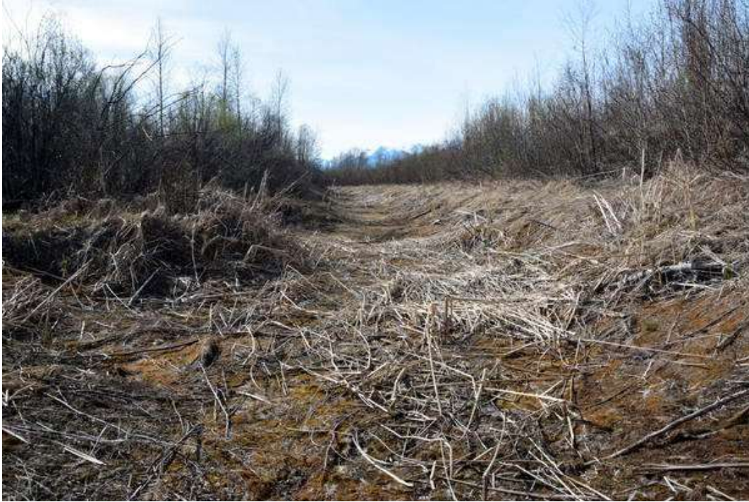
Figure 42. This deep and wide ditch was formed by the dragline when it removed soil for building the adjacent dike. The area where soil was removed is called a borrow pit, and this is a borrow pit ditch. The ditch moves surface water and groundwater downhill towards the water control structure. Water also soaks into the ground and flows under the dike into the Columbia River.
