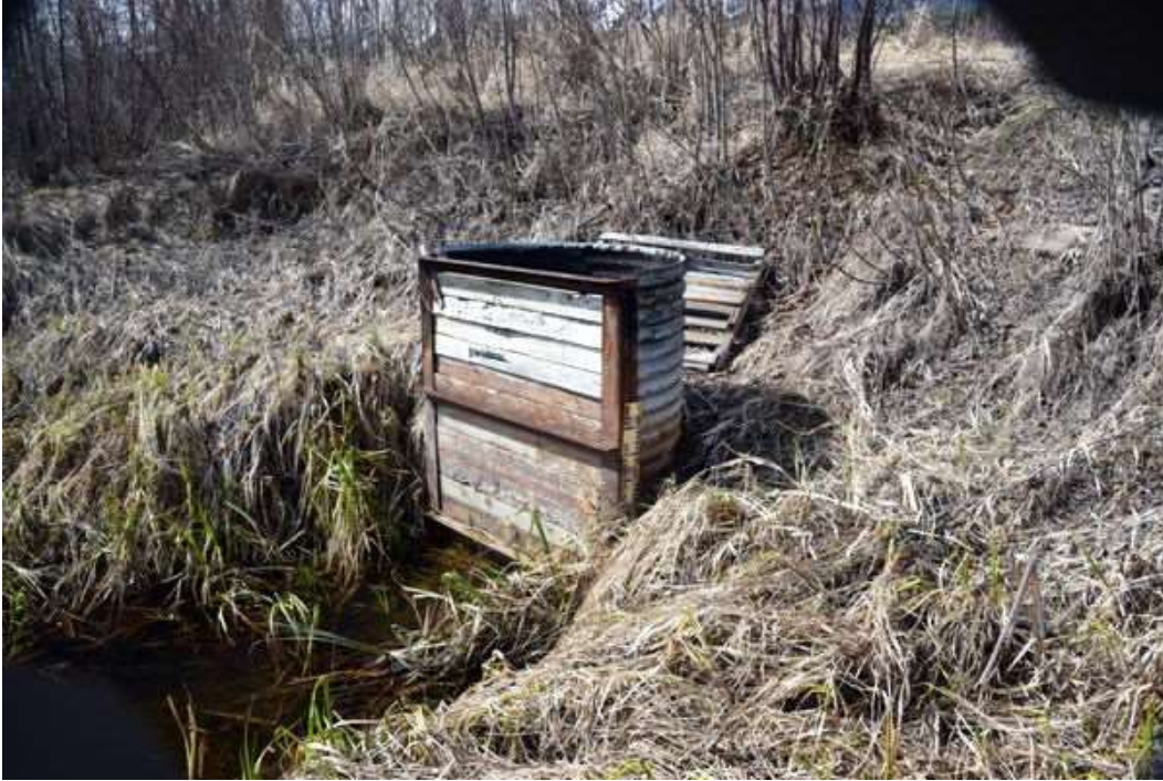
Figure 122. The flashboard riser and pipes for the Bergenham Compartment may be removed. Water levels would be near the top of the structure if the dike and water control structure were holding water.
