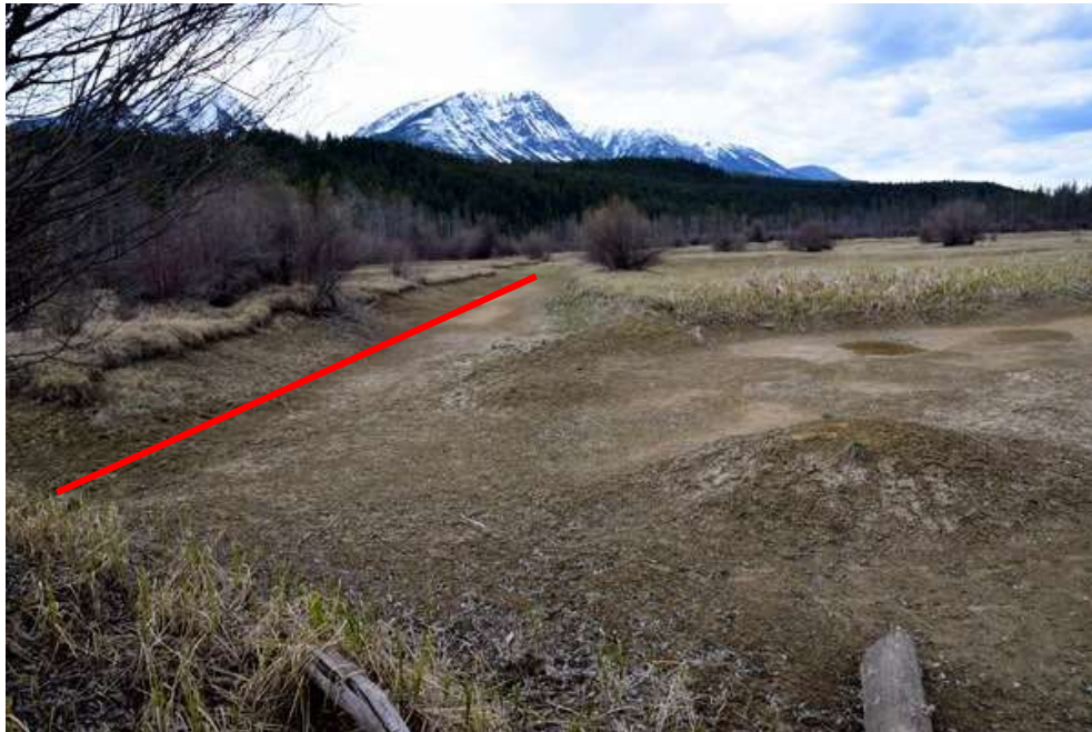
Figure 90. The borrow pit created by building the dike (red line) is draining the entire Northern portion of Moberly Marsh. Gravel lenses exposed in the ditch are carrying water under the dike into the Columbia River.
