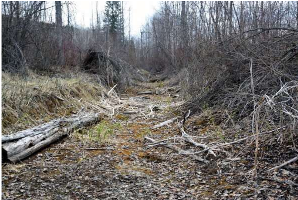
Figure 52. This photo shows where soil was removed to build a dike for the Bergenham Compartment. The area where soil was removed is called a borrow pit. Borrow pits parallel dikes, and slope downhill towards water control structures and pipes. The borrow pits formed ditches that are draining Moberly Marsh.
