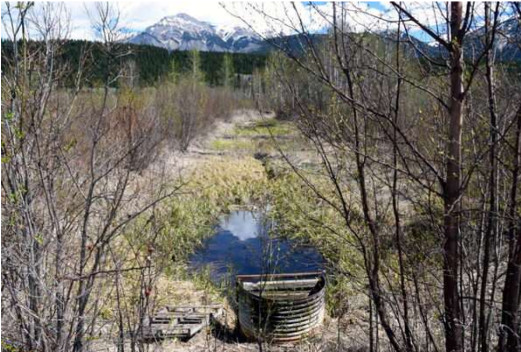
Figure 55. This long ditch was dug for the Bergenham Compartment as part of the 3-Way Control Structure. A flashboard riser water control structure was installed at the end of the ditch. The ditch was started before 1949, then deepened, widened, and lengthened after 1965. The flashboard riser and surrounding dike are leaking and not holding water. The elevation of water in the flashboard riser water control structure was the same as the elevation of water in the river. Removing water control structures, filling ditches, and restoring the elevation of natural levees along the Columbia River would restore water levels in Moberly Marsh.
