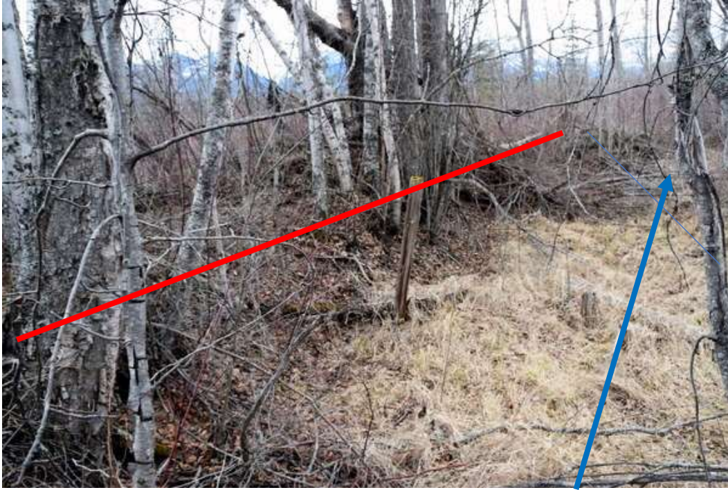
Figure 20. The red line marks a section of a dike built before 1965. The blue arrow marks a ditch dug at the same time. The dike was built using soil removed from digging the ditch, and helped prevent water from the Columbia River from flooding a portion of Moberly Marsh.
