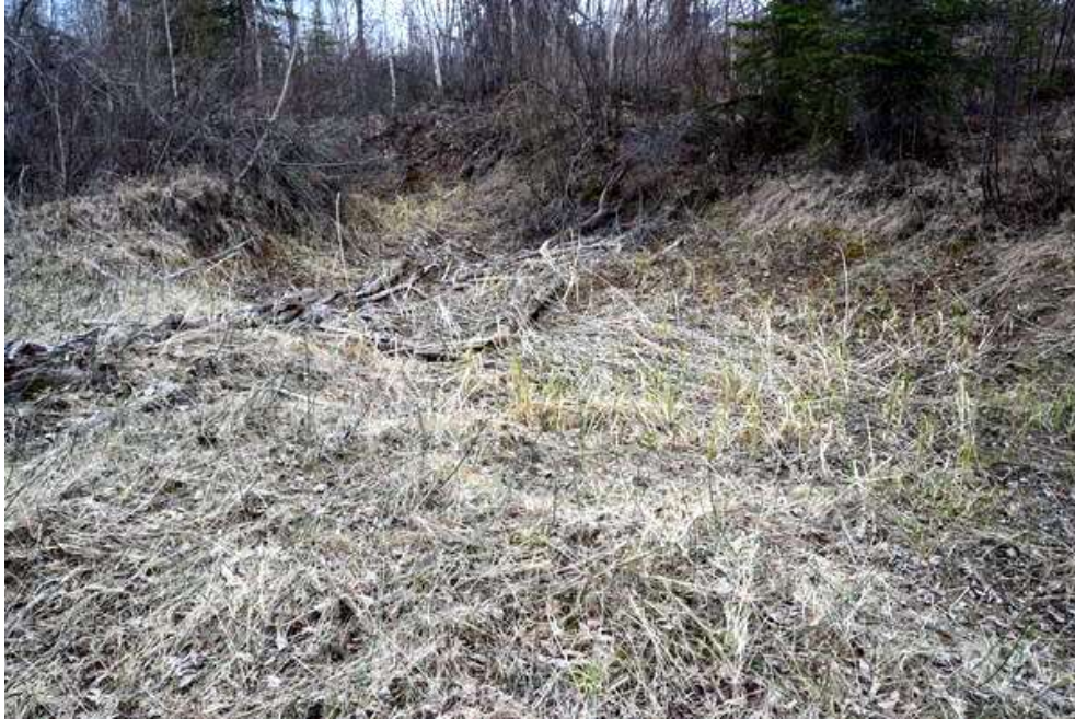
Figure 51. This drainage ditch was dug prior to 1965 near the Southern end of Moberly Marsh. The ditch was blocked by a dike built for the Bergenham Compartment. Water is soaking into the ground and flowing under the dike.
