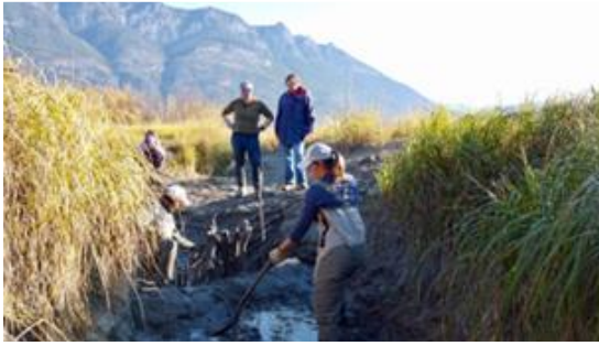
Volunteers helping with BDA construction in 2022.
